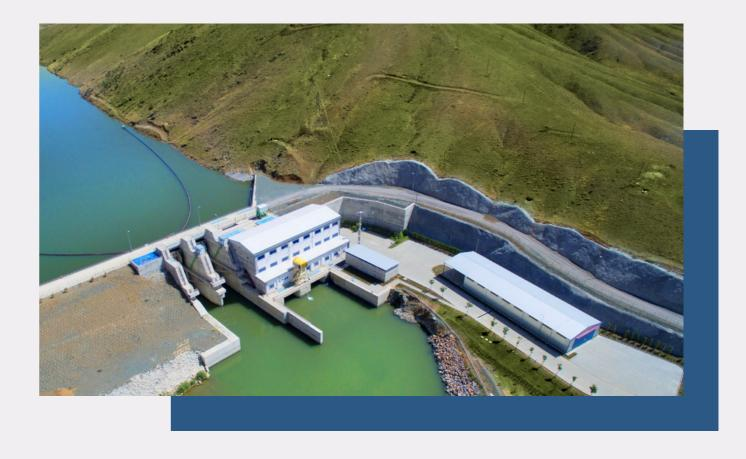
Starting operation in 2013, Çambaşı HEPP is located in Çaykara, Trabzon, on the Solaklı Stream. The plant has a 44-MW installed capacity with two separate regulators, a 2-km energy tunnel and two Pelton turbines with a 22.05-MW capacity.
