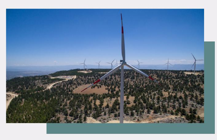
Starting operation in 2012, Dağpazarı WPP is located in Mut, Mersin, and has an installed capacity of 39 MW with 13 turbines. The project was awarded the "Carbon Gold Certificate" by The Gold Standard Foundation.
