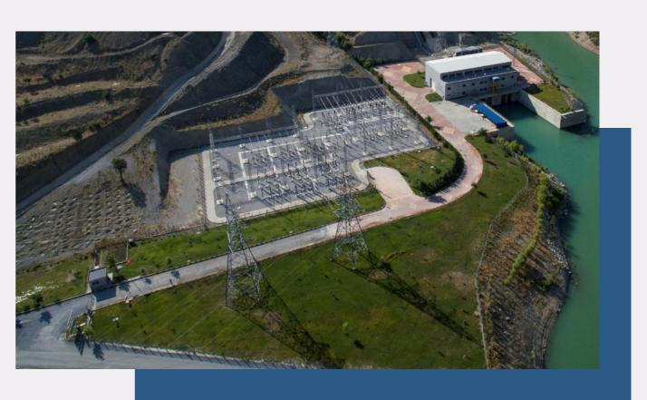
Starting operation in 2011, Hacınınoğlu HEPP is located in Kahramanmaraş, in the Ceyhan Basin. The plant is connected to TEİAŞ' Kılavuzlu and Narlı switchyard of 154 kV, and has an installed capacity of 142 MW.
