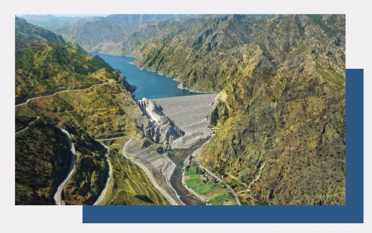
Starting operation in the second quarter of 2014, Arkun HEPP is located on the Çoruh River on the provincial border of Erzurum-Artvin. The plant's total installed capacity is 245 MW with three main turbines with a 78-MW capacity and two environmental flow plants with a 5.4-MW capacity.
