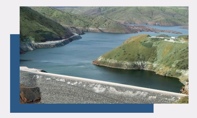
Starting operation in 2014, Kandil Dam and HEPP is located in Kahramanmaraş, in the Ceyhan Basin. The project, which includes a rock fill dam with a concrete-covered front, has a total installed capacity of 208 MW. Its two Francis turbines have a 102-MW capacity and its single environmental turbine has a 4-MW capacity.
