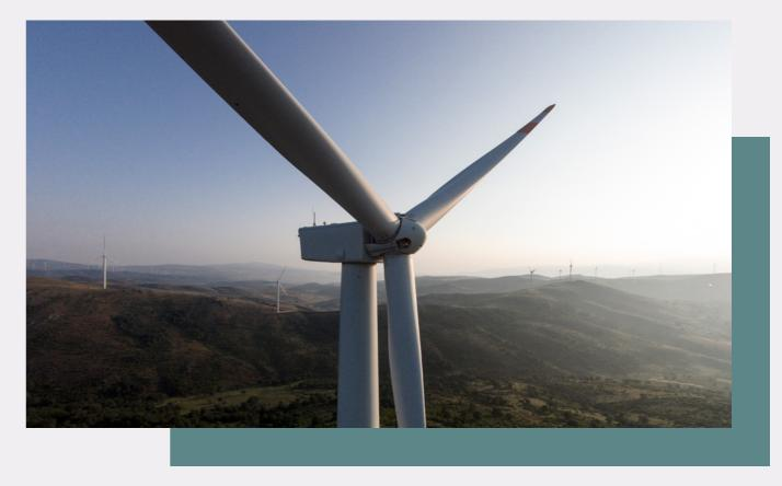
Starting operation in 2013, Balıkesir WPP is located in Balıkesir and has a capacity of 143 MW with 52 turbines. The plant is connected to the TEİAŞ' Poyraz and Balıkesir 154-kV switch. The project was awarded the "Carbon Gold Certificate" by The Gold Standard Foundation.
