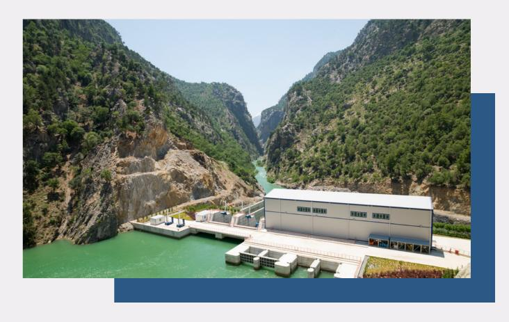
Starting operation in 2013, Köprü HEPP is located in Adana, on the Göksu Bayou of the Seyhan River. The dam has an RCC body and twin Francis turbines, each with a 78-MW capacity. Its total installed capacity is 156 MW.
