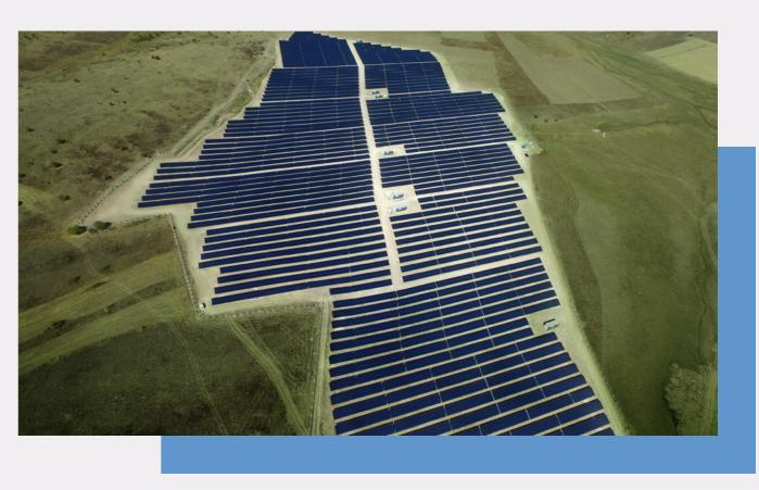
Starting operation in 2017, Karabük SPP is located in Bölükören, Eskipazar, Karabük. Built on 140-acre land, the plant includes solar panels that employ PV thin-film technology.
