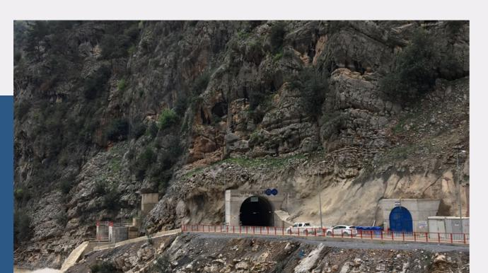
Starting operation in 2017, Doğançay HEPP is located in the Seyhan Basin, Adana, on the Doğançay Creek. This plant, which has a capacity of 62 MW, is built using a tunnel boring machine (TBM) instead of traditional methods. All of the plant's units are subterranean, except for the regulator area.
